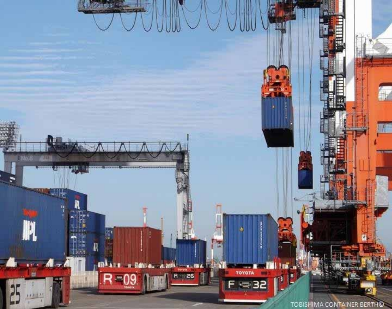
TOBISHIMA CONTAINER BERTH ©
